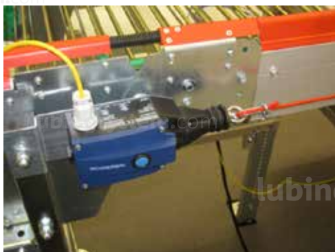
Installation on drive unit
