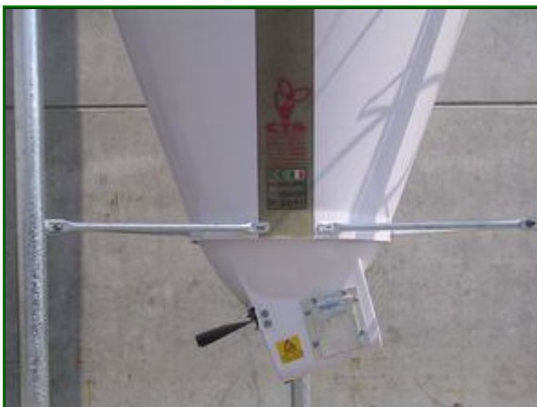
Code C5 Silos well. Unloading using a flexible screw conv. inclination of 20° with shutter for feed. D:780mm H:700mm
