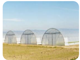
Air pre-heated by solar energy
