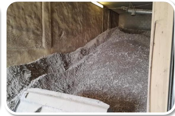
Concrete bunker: low budget intake bunker
